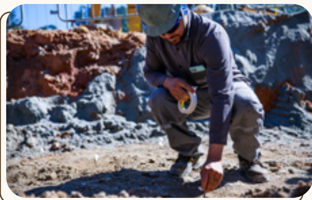
Obra Scala data centers - Barueri, SP
